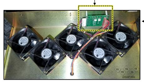
NORTEL NT3X90AF, DMS-100 SWITCH BAY (DC POWERED) w/ EXISTING FANS (5 FANS PER TRAY)
