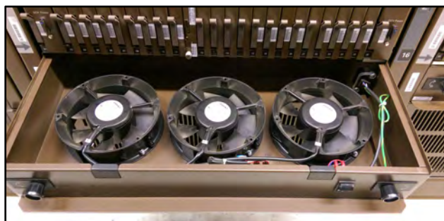
DMS-100 NTRX91AA FAN UNIT w/ EXISTING FANS
