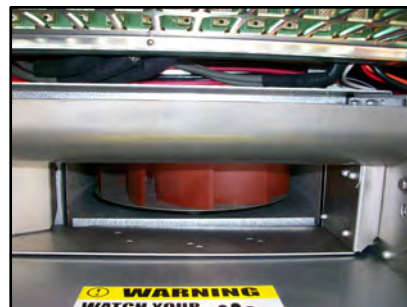
BOTTOM OF MESA CABINET w/ EXISTING FAN (ORDER UPN # TF-MC225-02)
