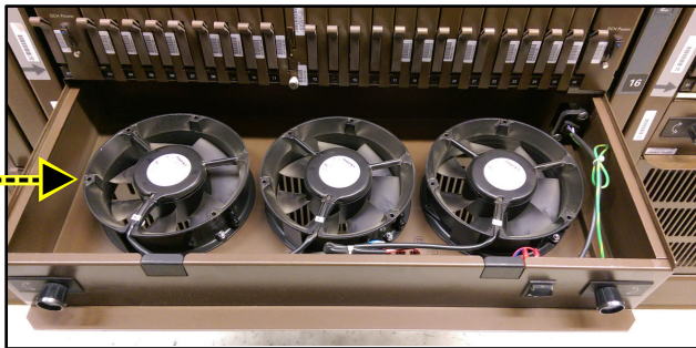
DMS-100 NTRX91AA FAN UNIT w/ EXISTING FANS
