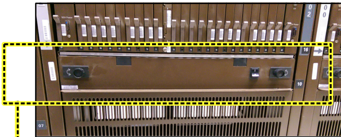
DMS-100 NTRX91AA FAN UNIT w/ EXISTING FANS
