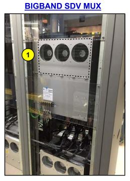
**5.** Remove the remaining (8) screws & washers attaching the existing guard grills & fans to the fan tray.
