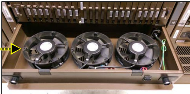
DMS-100 NTRX91AA FAN UNIT w/ EXISTING FANS
