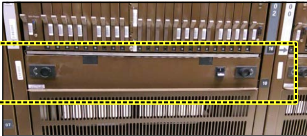
DMS-100 NTRX91AA FAN UNIT w/ EXISTING FANS
