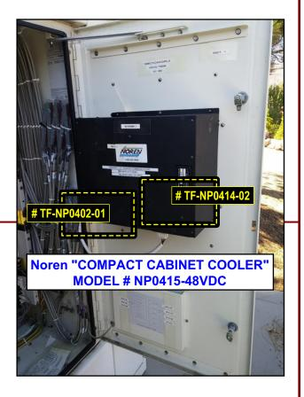
PN # TF-NP0414-02 48 Volt Replacement Heat Exchanger for Noren Cooling Unit - External (8.45K)
