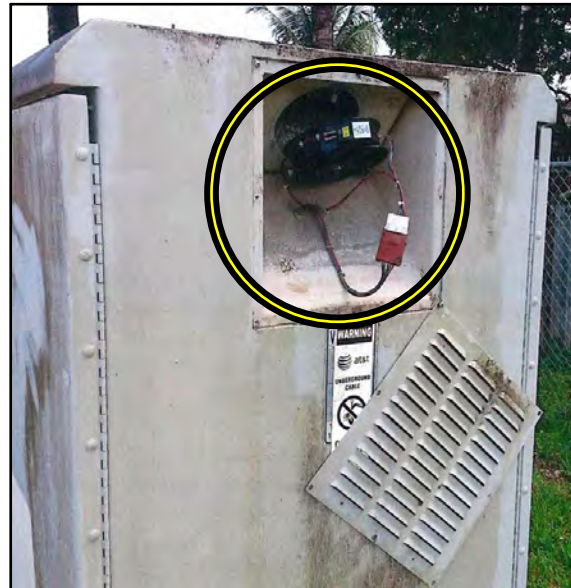
PN # TF-FUJ6200-01 48V Replacement Heat Exchanger for Fujitsu 6200 Cabinet w/ 5 Wire Plug
